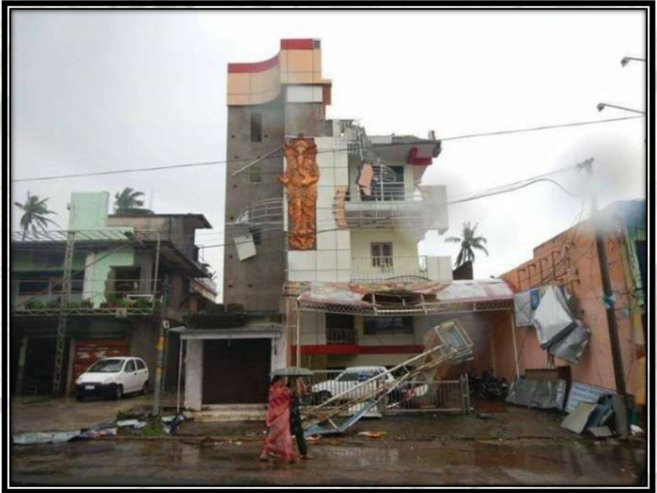
Phailin damage in Berhampur
